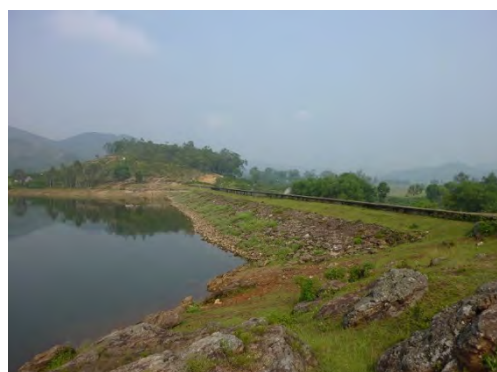
Photo 6: Ho Thanh reservoir (countermeasure to reservoir leakage was taken from the center to the right-hand side of the photo)
