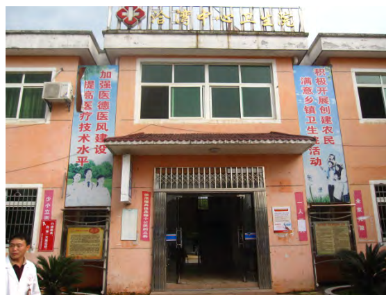
Township hospital where immunization is conducted (Nanfeng County, Jiangxi Province)
