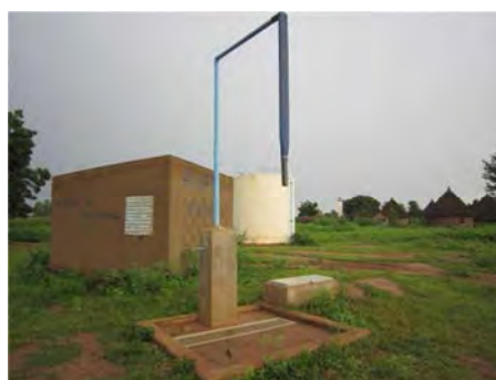
Newly constructed watering place for vehicle in Goumbayel
