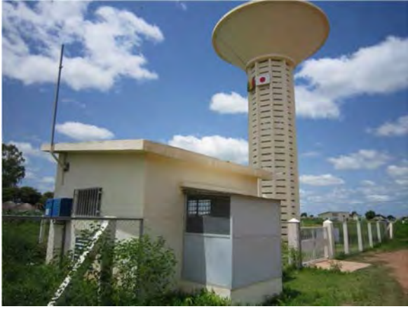
One of the renovated water supply facilities in the target sites, Sinthiou Maleme
