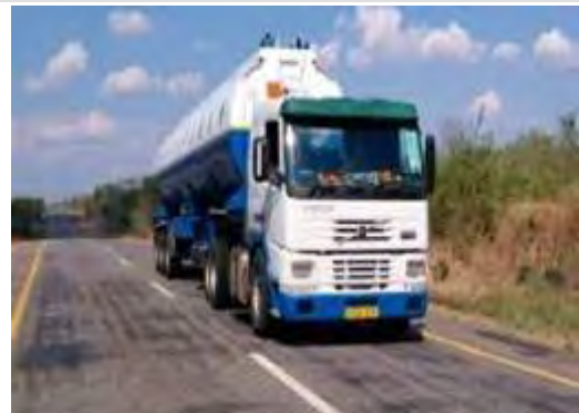
Vehicle on Section of Road Covered by the Project
