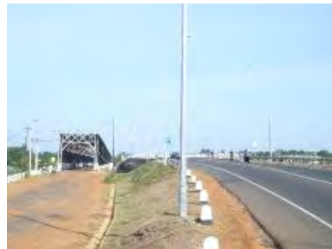
Kallady Bridge (Left bridge is an old bridge) (Picture provided by Oriental Consultants Co., LTD)
