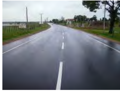
National Road A15 at Trikkandimadu After project
