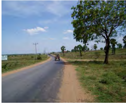
National Road A15 at Trikkandimadu Before project
