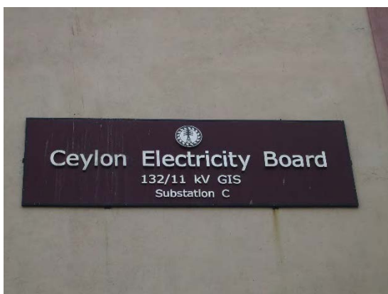
Entrance of Substation “C”
