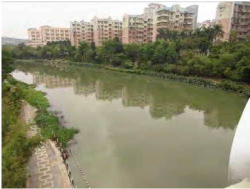
Photo 2: A revetment built on the Zhupaichong Stream
