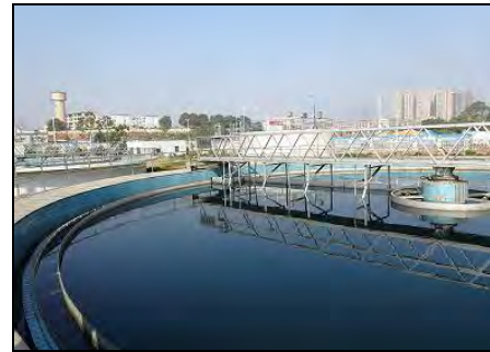
Photo 2: Liaojia Citang Water Purification Plant
