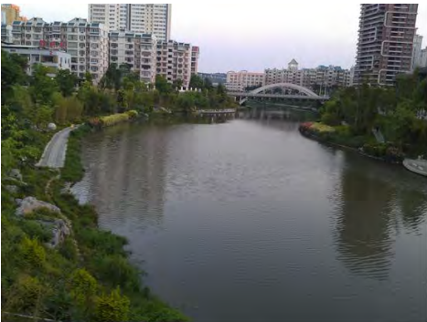
Photo 1: In Nanning city, revetments and bridges were constructed
