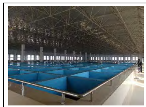
Photo1: A Purification Plant Built with This Project
