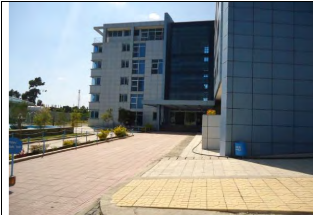
Photo-1 Federal EWWCE
