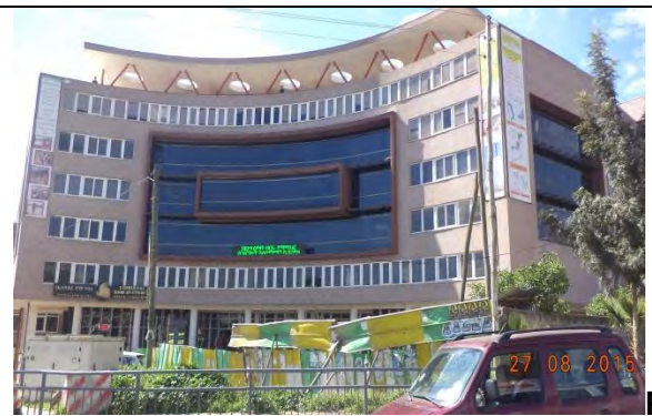
Photo-6 Addis Ababa Federal WWDSE
