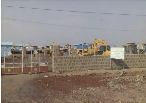
Photo-1 Semera Water Works Construction Enterprise Workshop
