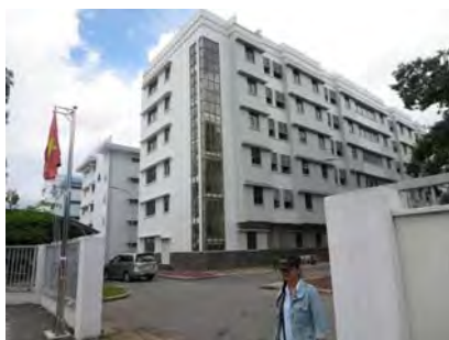
SADECO Apartment Building
