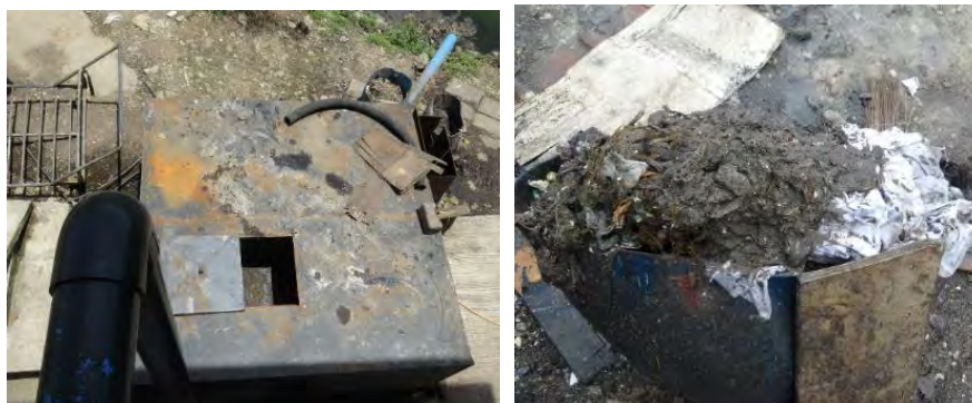
Photo: Septage receiving tank temporarily placed to remove solids in septage and removed solids
