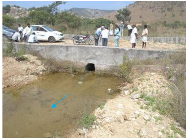
(Left Main Canal) Off take 1: Reconstruction
