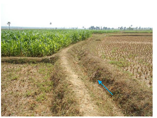
Field channel : Reconstruction
