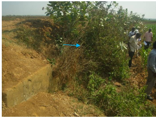
Surplus Weir 2 : Reconstruction
