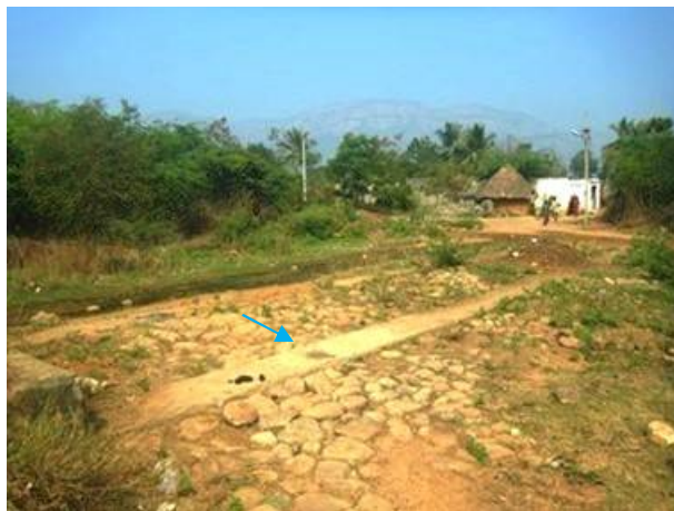
Surplus Weir : Reconstruction
