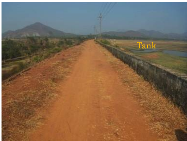
(Dam) Top of Bund (Dam): Repair
