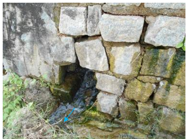
(Right Main Canal) Aqueduct: Reconstruction
