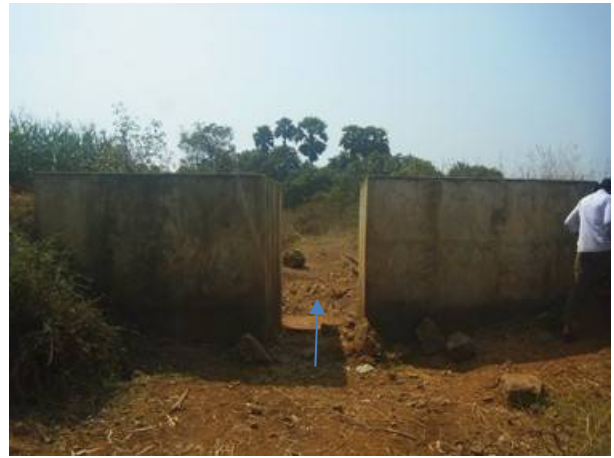
(Left main canal) Regulator: Replacement of gate
