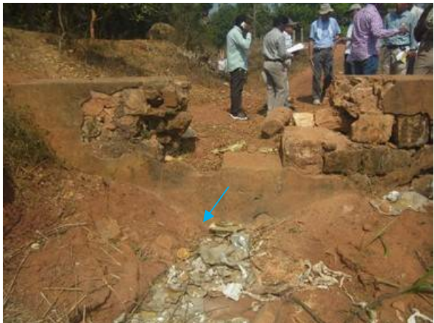
(Left main canal) Drop: Reconstruction
