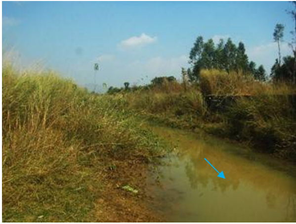
Right Main Canal: Lining
