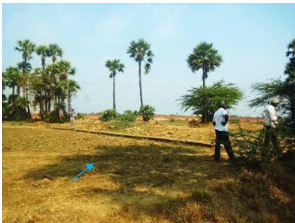
Surplus Weir 2 : Reconstruction
