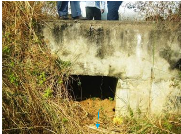
Right Main Canal: Distributor_UT (Drain Syphon)
