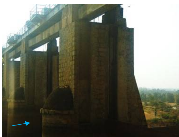
(Spillway) Gates: Replacement (wire ropes, rubber seals, painting etc.)
