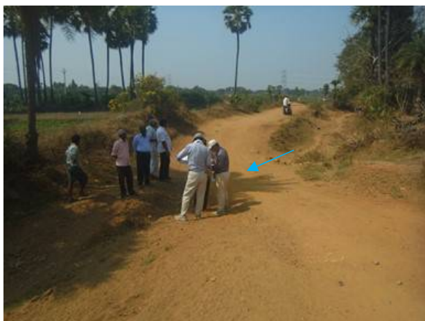
Feeder canal : Reconstruction
