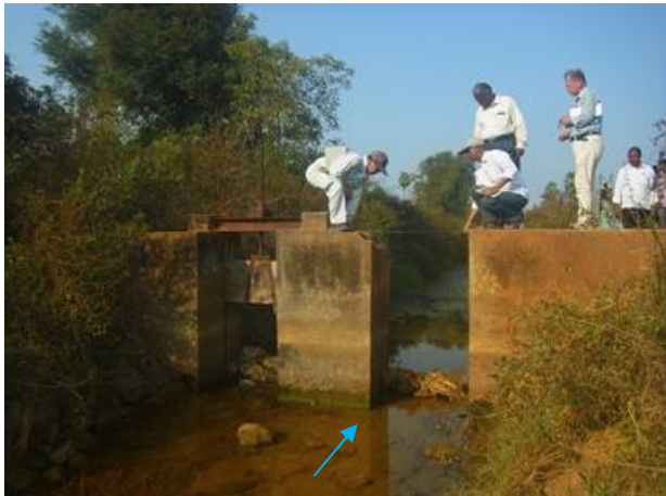
(Right main canal) Regulator: Reconstruction
