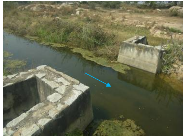
(Left Main Canal) Under Tunnel (Syphon): Reconstruction
