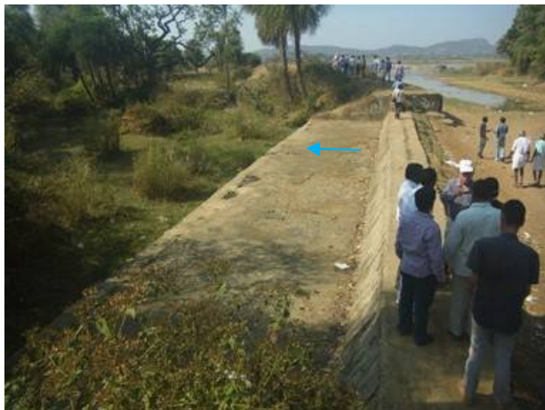
Surplus weir : Reconstruction
