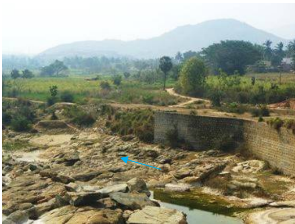
(Spillway) Eplon: Repair
