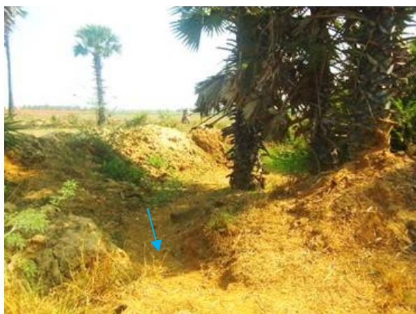
Feeder canal : Reconstruction
