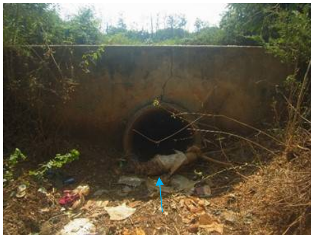
(Left main canal) Siphon: Reconstruction
