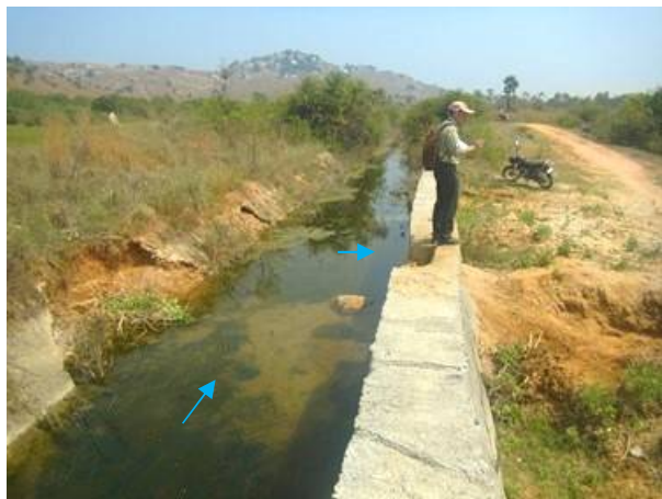
(Left Main Canal) Off take 1: Reconstruction
