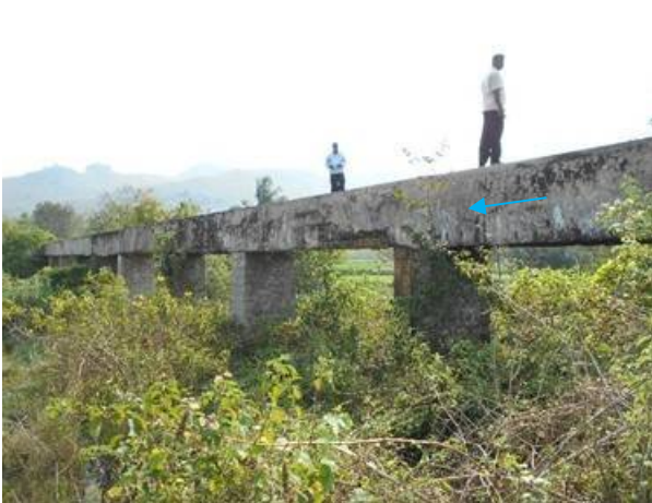
(Right Main Canal) Aqueduct: Reconstruction
