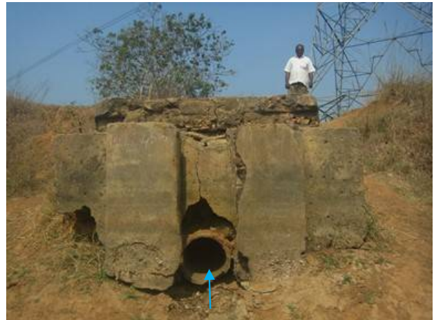
(Left main canal) Off take: Reconstruction
