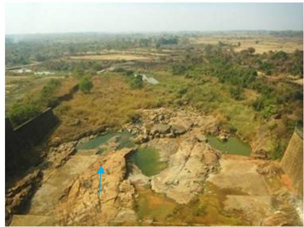
(Spillway) D/S apron: Repair
