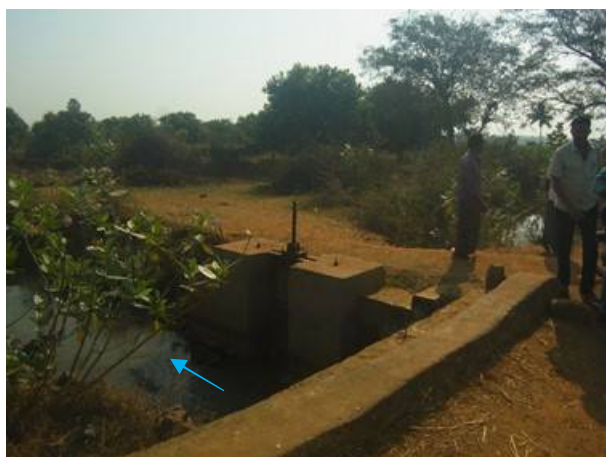
(Monkollu main canal) Off take: Wall type canal
