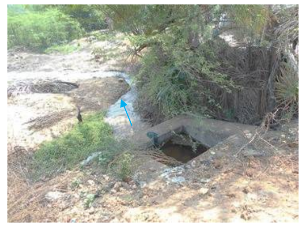
Supply canal 2 : Reconstruction
