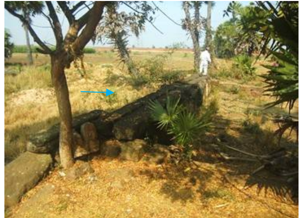
Surplus Weir 1 : Reconstruction
