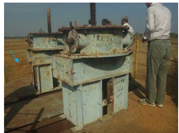
(Left side intake) Gate: Replacement
