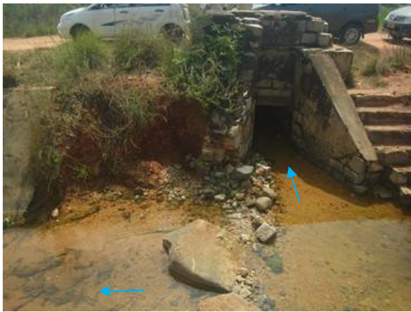
(Left Main Canal) Off take 2: Reconstruction
