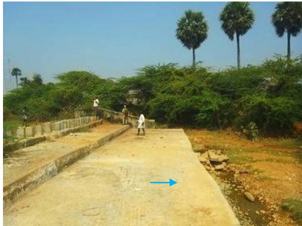
Surplus Weir : Reconstruction
