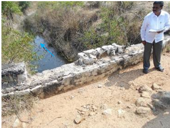
(Left Main Canal) Super Passage: Reconstruction
