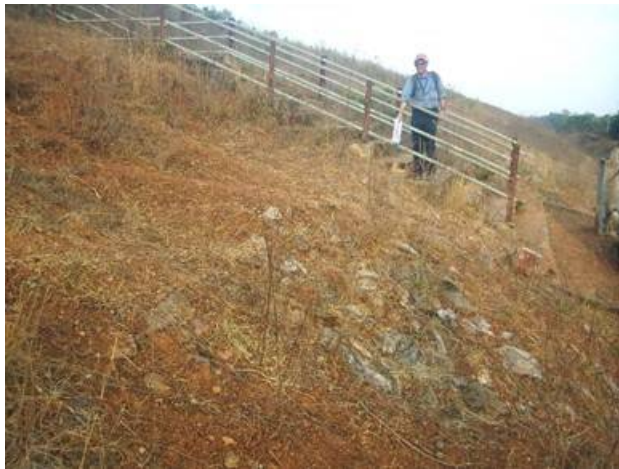
(Dam) Toe drain: Repair
