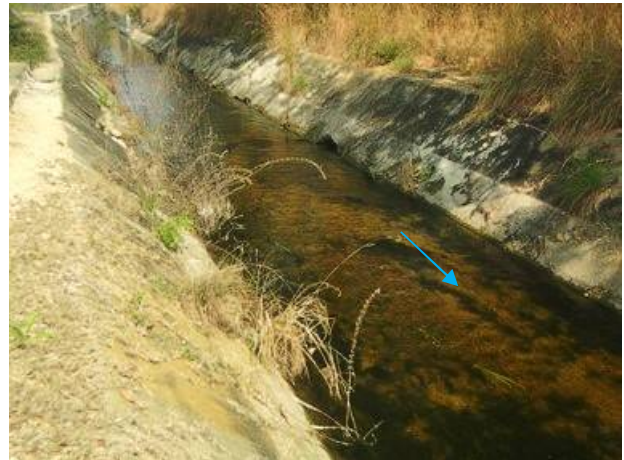
(Left Main Canal) Concrete Lining: Reconstruction
