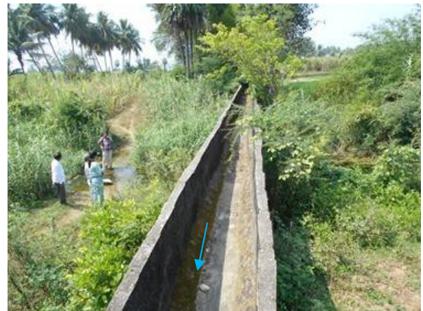
(Left Main Canal)_Aqueduct: Reconstruction
