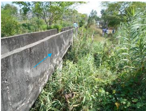
(Left Main Canal)_Aqueduct: Reconstruction
