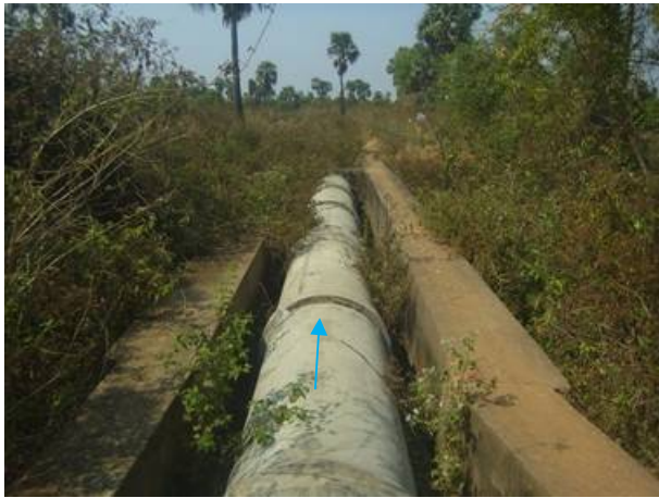
(Left main canal) Aqueduct: Reconstruction
