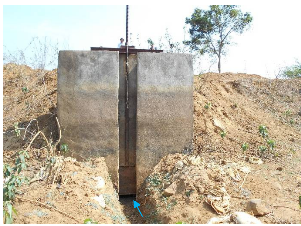
Gate of sluice : Replacement
