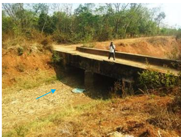
Right Main Canal: Distributor_Bridge
