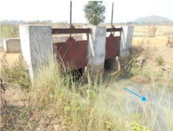
Right Main Canal: Regulator and Bridge
