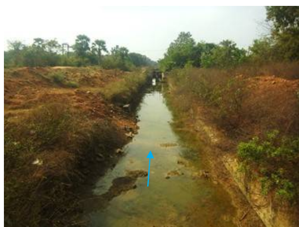
(Left Main canal) Wall type canal: Reconstruction
