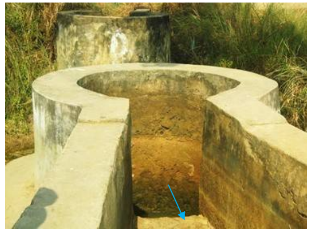
Right Main Canal: Distributor_Syphon
