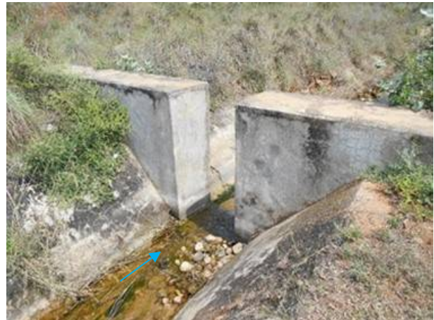
(Left Main Canal) Drop: Reconstruction
