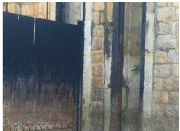
(Spillway) Rubber seals of gates: Replacement
