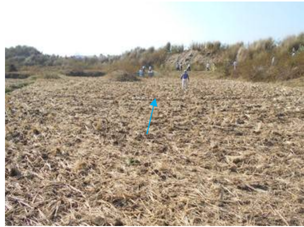
Surplus Weir : New construction
