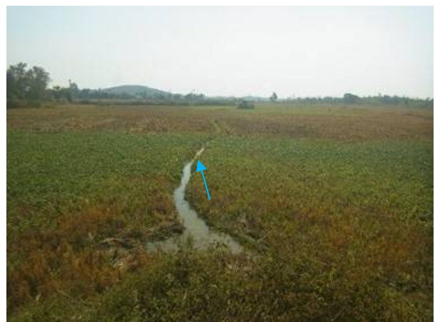
Field channel : Repair
