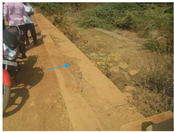
Surplus Weir 1 : Reconstruction
