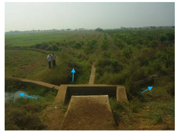
Field channel : Reconstruction
