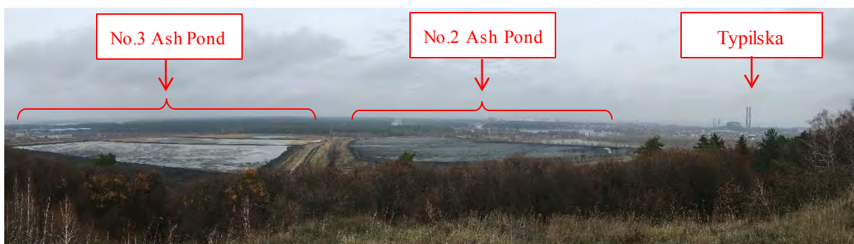
Figure 5.2-3 Distant view of Ash pond from south
