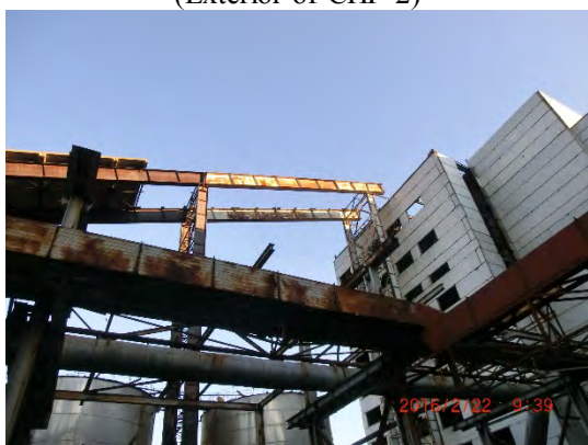
(Conveyer installed halfway)
