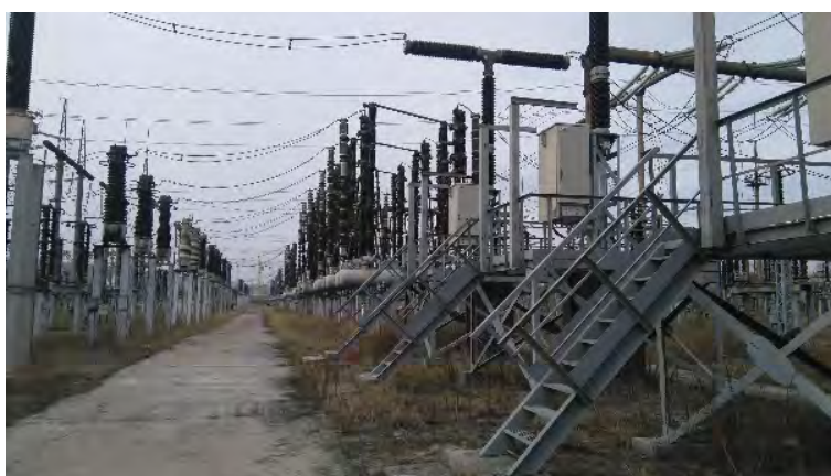
Figure 5.2-7 Condition of Switchyard
