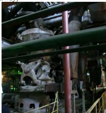
(Coal pulverizer installed)
