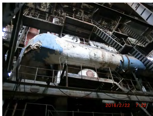
(Boiler made by Mitsubishi)
