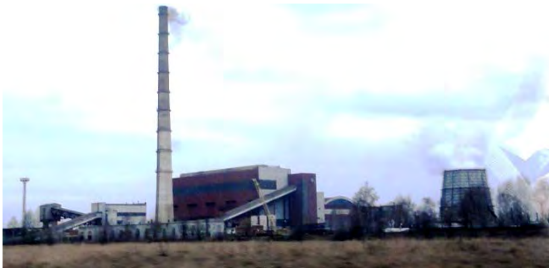
(Exterior of Kaluska CHP (currently, No.2 is in operation, No.1 inspected and No.3 and 4 suspended))
