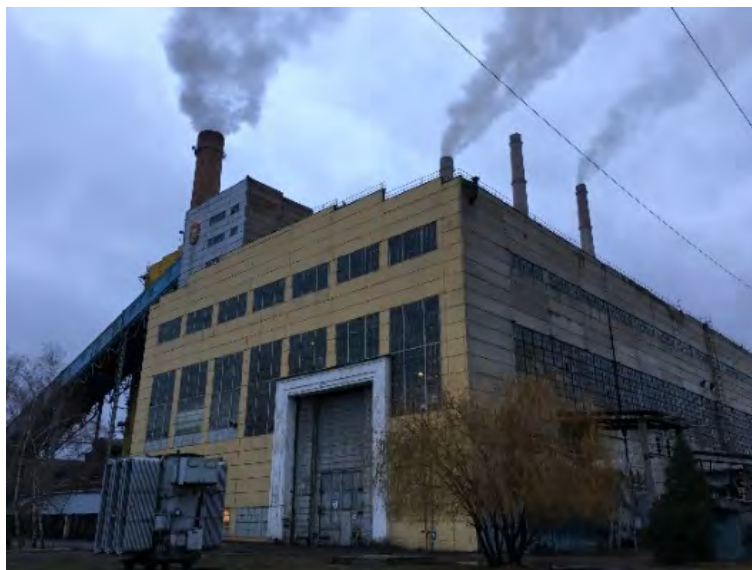
Figure 5.2-11 Smoke from chimneys (yellow-colored flue gas was seen)
