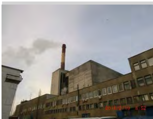
Figure 8.1-3 Exterior of the Enerzia waste incineration plant
