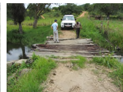
Photograph-8: Wooden bridge checking in GC07
