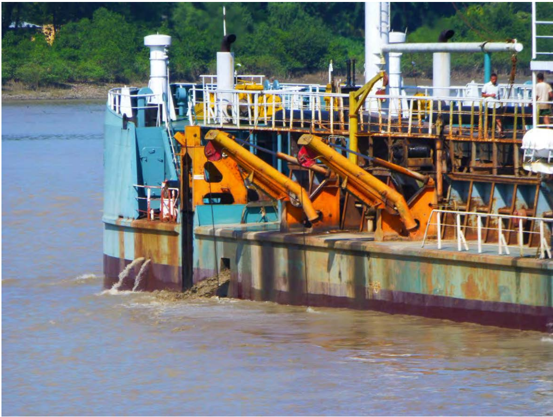
13. Operation of Dredging
