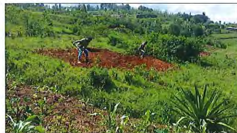
Backfilling of the borehole
