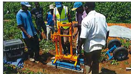
Installation of the base
