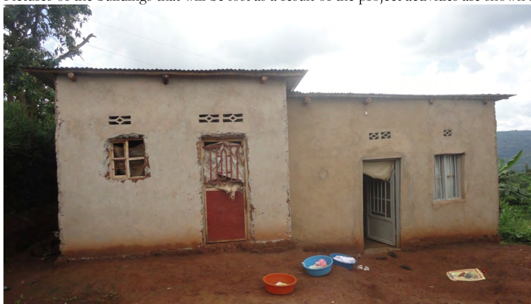
Figure 3: One of the buildings in Bumbogo Sector that will be affected by Project
