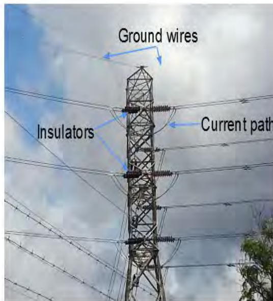
Figure 3: An example of components of a tower
