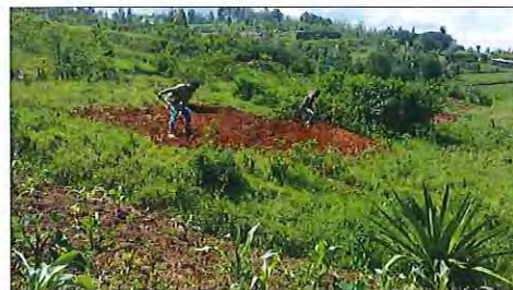
Backfilling of the borehole
