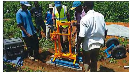
Installation of the base
