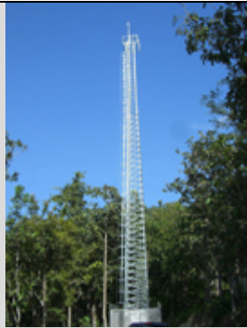
Completed tower for WiMAX
