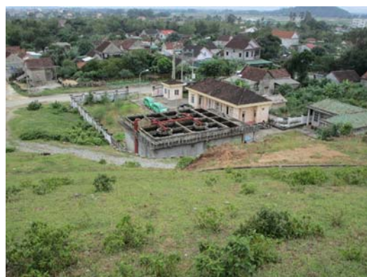
Water Purification Plant in Viet Nam (Khe Doc Water Purification Plant)
