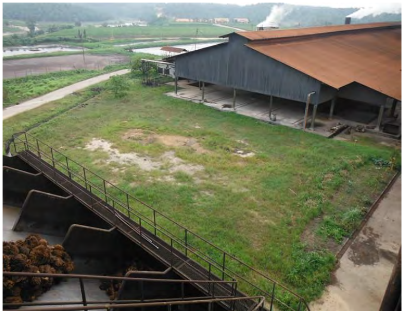
Pilot Plant Construction Site
