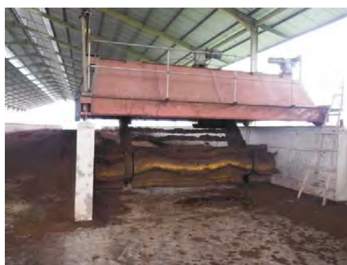
Survey of the scoop type composting facility
