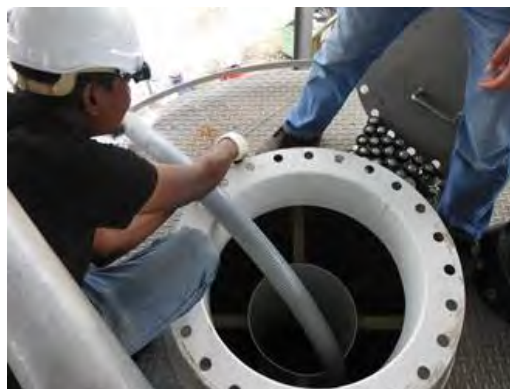
Transfer of Anaerobic Seed Sludge
