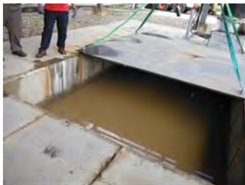
Leaching Ground Water into the System
