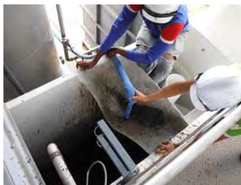
Transfer of Aerobic Seed Sludge
