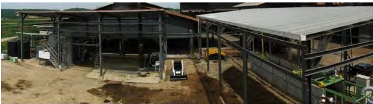
After construction of the Pilot Plant
