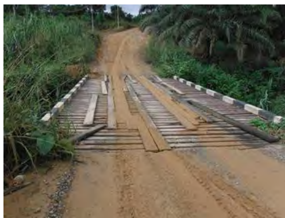
Simple bridge on the unpaved road
