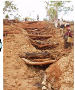
Erosion control with wattles
