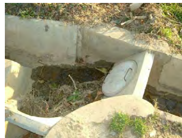
Assembly at site
