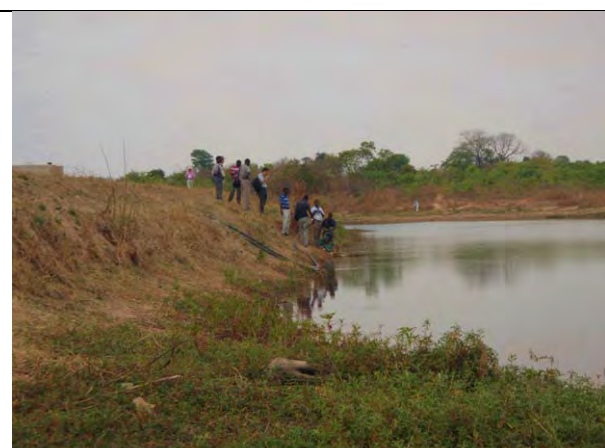
Members of the farmers' group are inspecting inlet of pipes, which are connected to a siphoning box on the bank.
