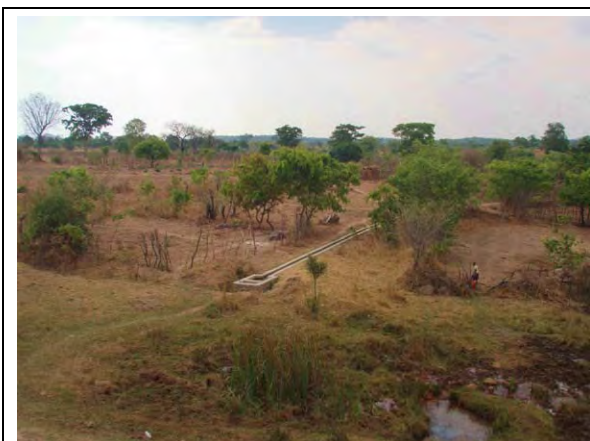
View of garden area from the bank side. Canal conveys water up-taken by siphon system to gardens in downstream direction.
