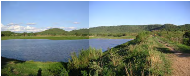
Chipapa Irrigation System (Kafue District) Reservoir and dam body
