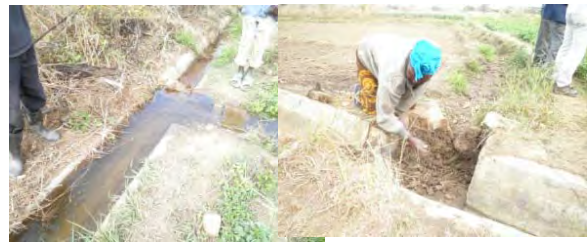
Irrigation canal and division pit Water is diverted by closing with earth materials.
