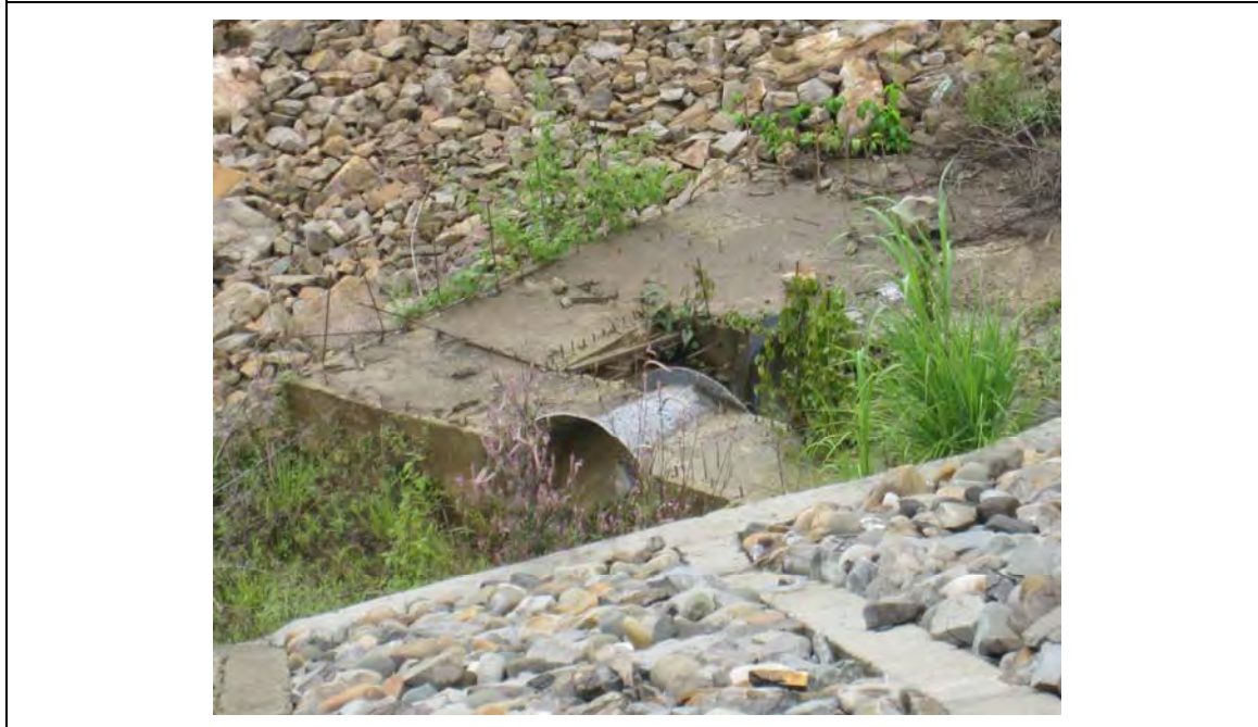
Low Intake Mouth of Raw Water in the Thoubal Dam
