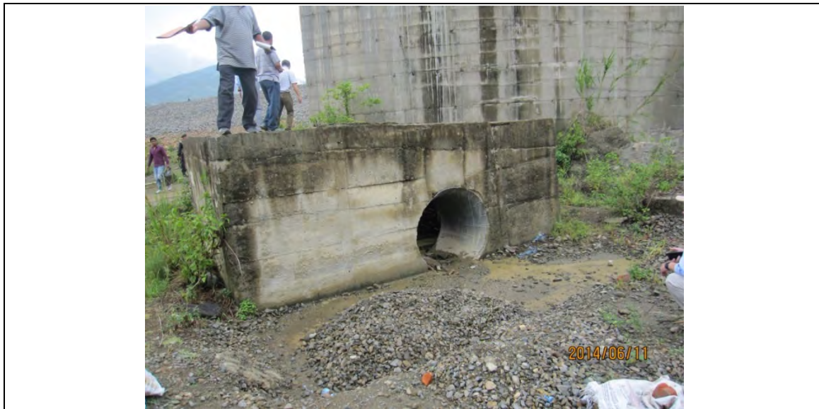
Upper Intake Mouth of Raw Water in the Thoubal Dam
