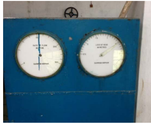
Photo 2.7 A loss of head gage for Rapid Sand Filters at Singda WTP
