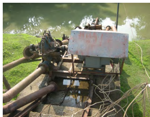
Photo 2.1 Raw Water Pump at Irilbung Intake
