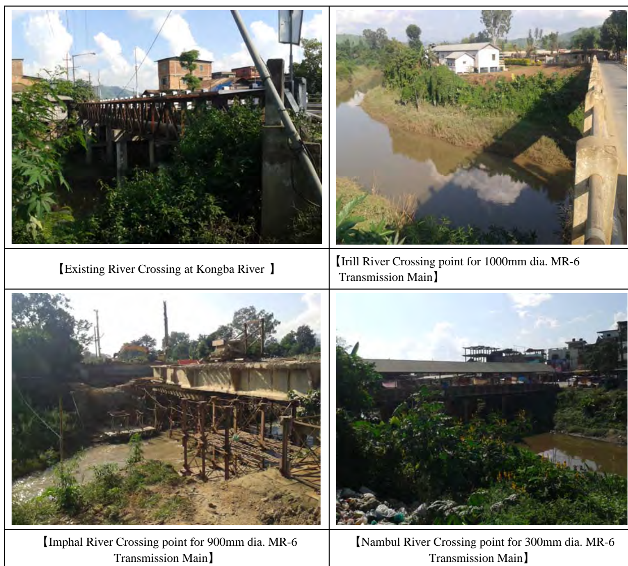
Photo 5.10 Existing Pipe Bridge and River Crossing Points for New Transmission Mains
