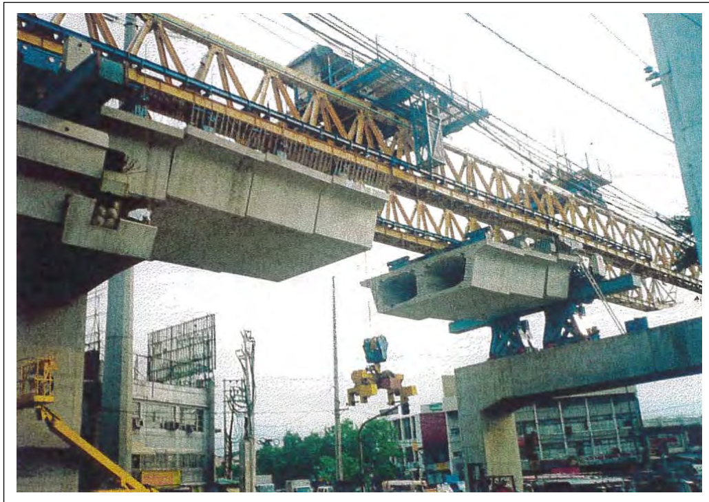
Photo 5.1-3 PC Box Girder Erection – LRT Line 2 (Truss Type Erection gantry)
