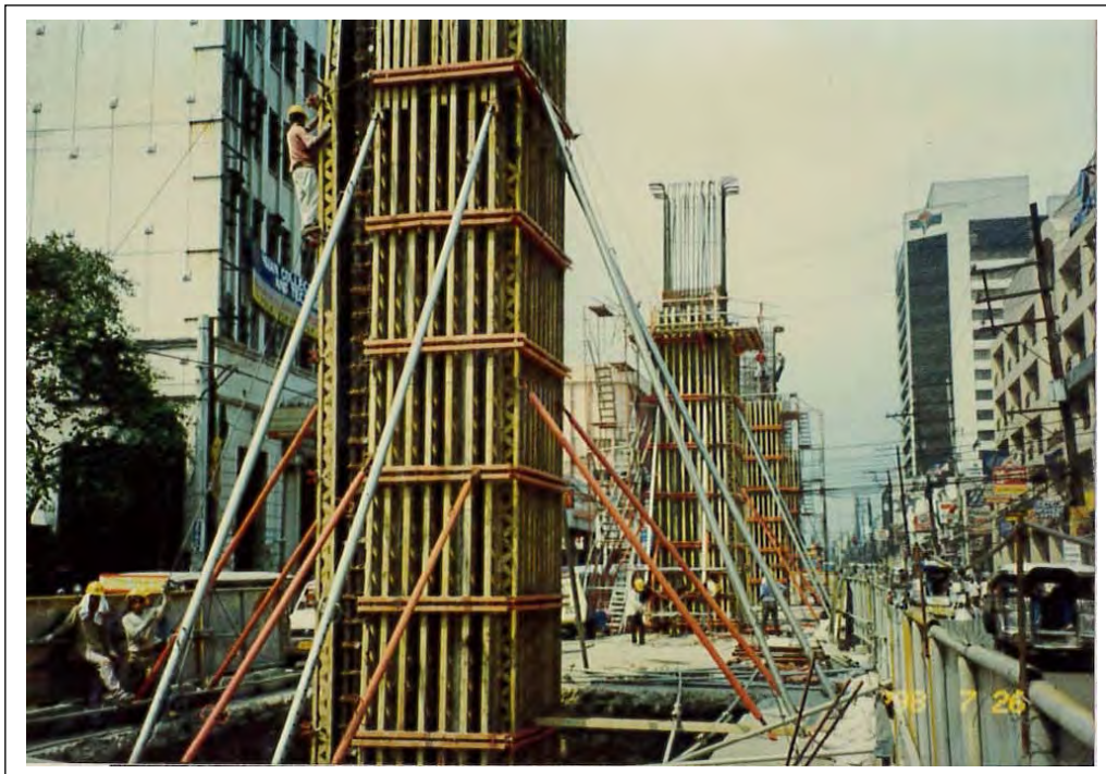
Photo 5.1-1 Pier Column Construction – LRT Line 2
