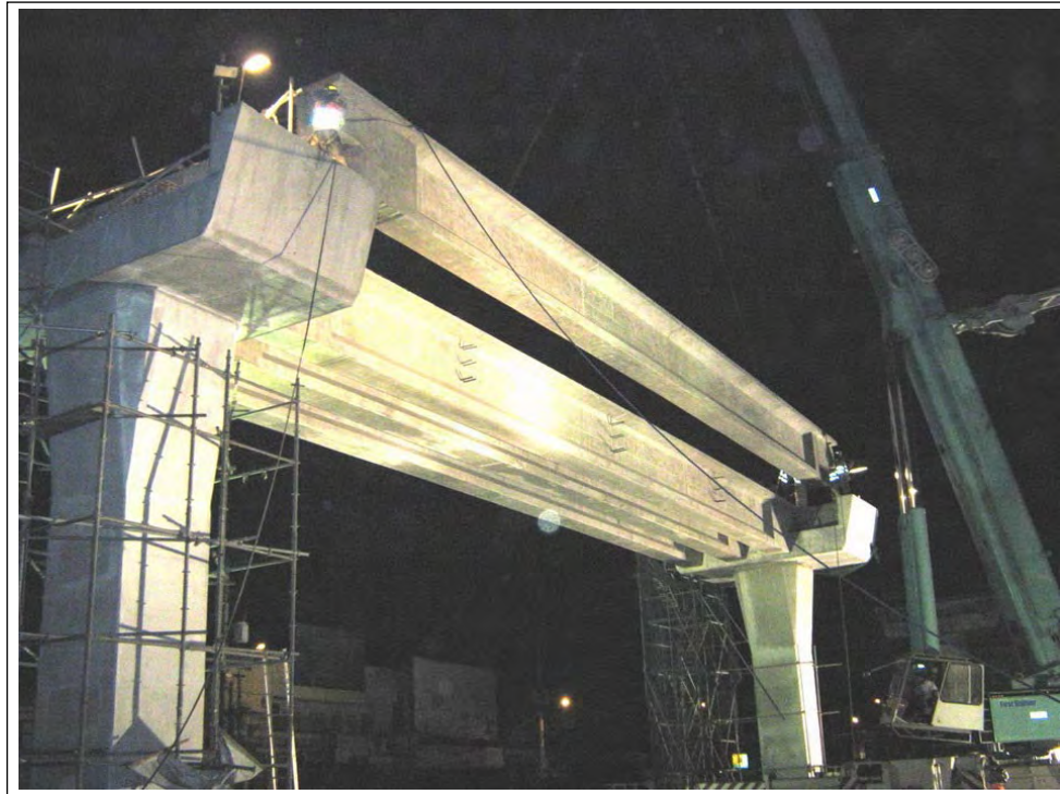
Photo 5.1-5 Girder erected at night by single truck mounted crane – LRT Line 1 NEP
