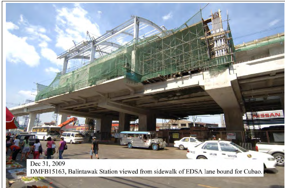
Photo 5.1-8 Station Platforms and Roof Frame under Construction – LRT Line 1 NEP
