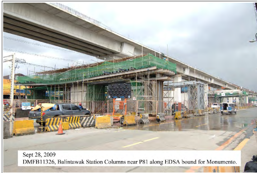
Photo 5.1-6 Station Cantilever Pier Construction – LRT Line 1 NEP
