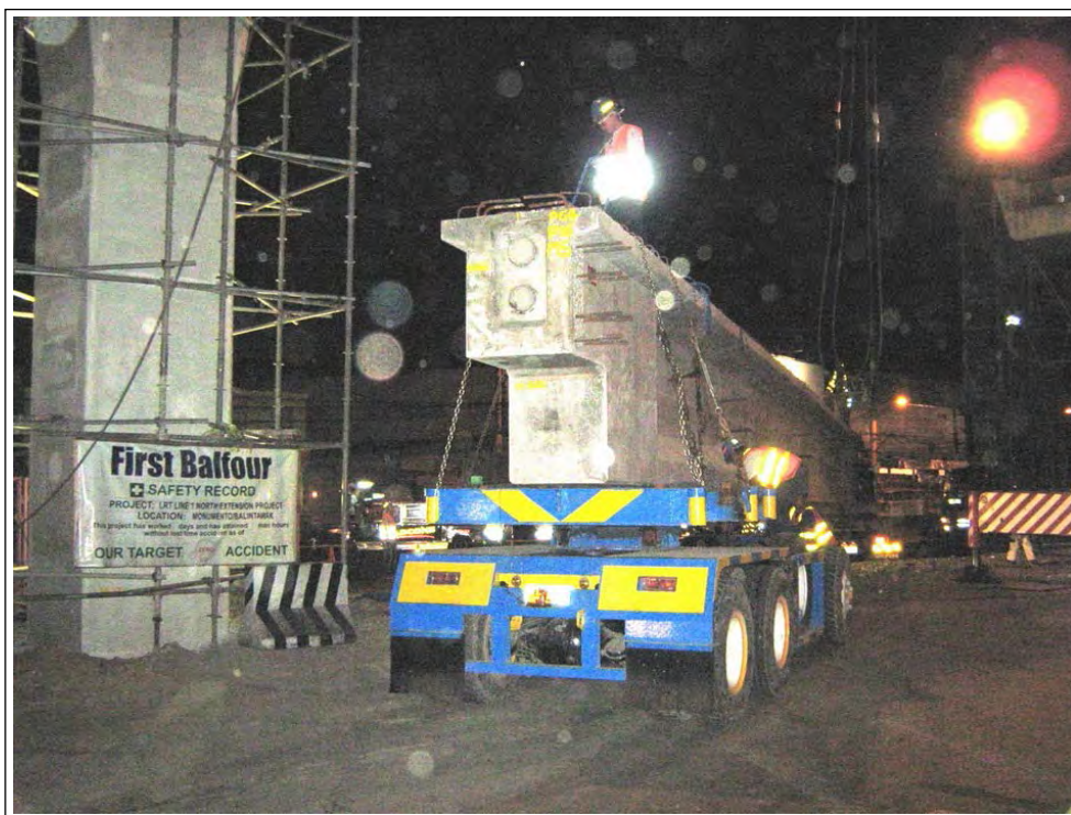
Photo 5.1-4 Girder delivered at night by trailer – LRT Line 1 NEP
