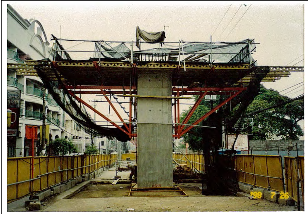
Photo 5.1-2 Pier Column Construction – LRT Line 2
