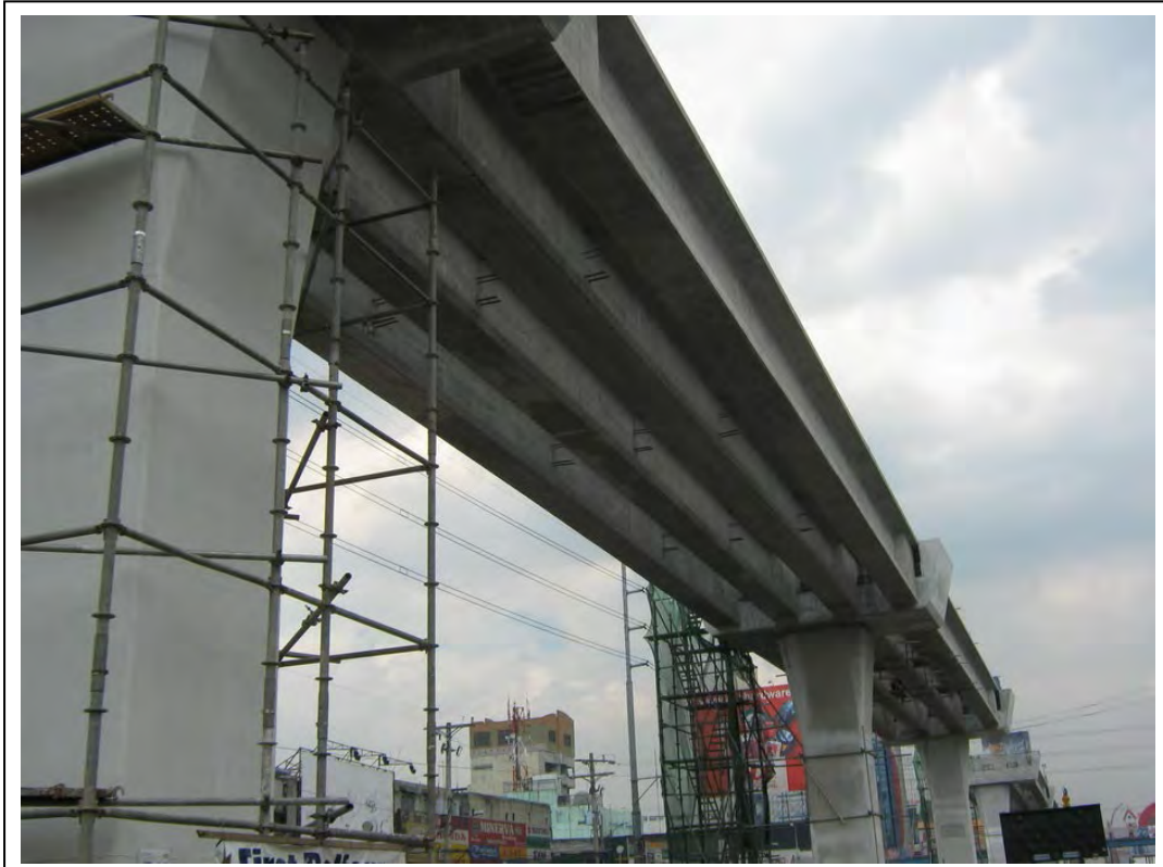
Photo 3.7-2 AASHTO Girder - LRT Line 1 NEP Girder – Manila
