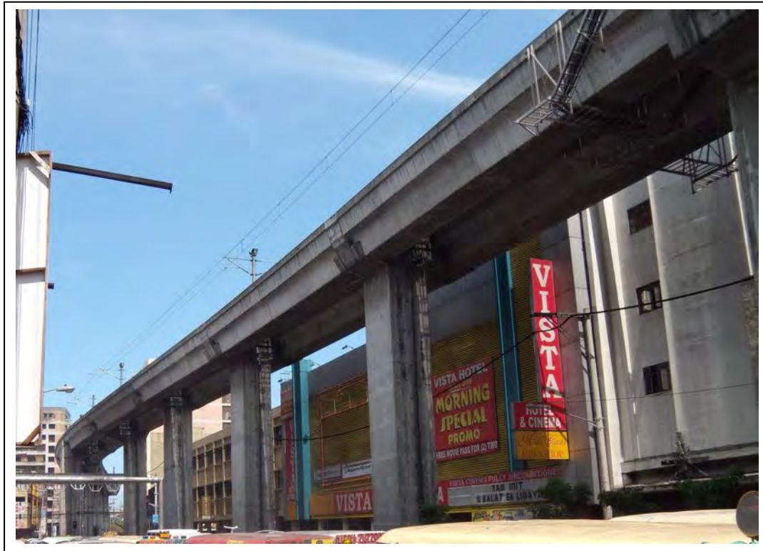
Photo 3.7-1 PC Box Girder - Existing LRT Line 2 Girder – Manila
