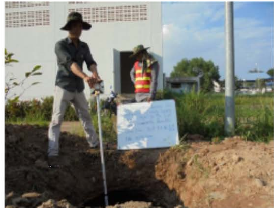
Test Pit No.4(300DIP Pipe found)
