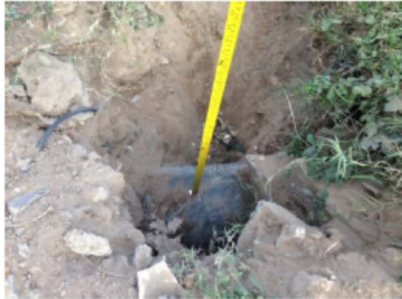
Test Pit No.14 (300 DIP Pipe found)
