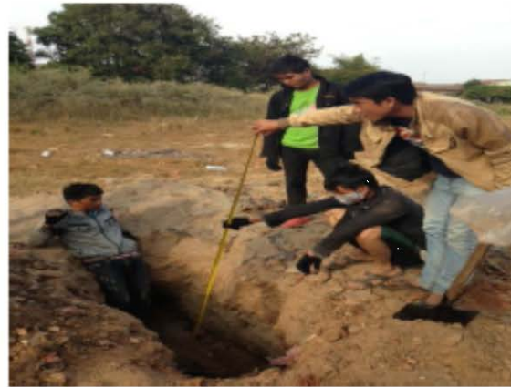
Test Pit No.16 (Pipe not Found, Over 2m-Dept)
