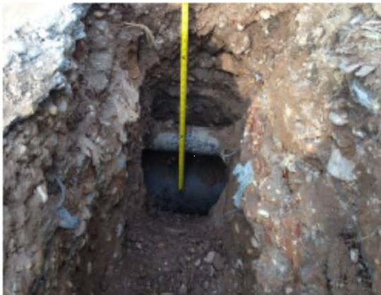
Test Pit No.11 (250DIP Pipe found)
