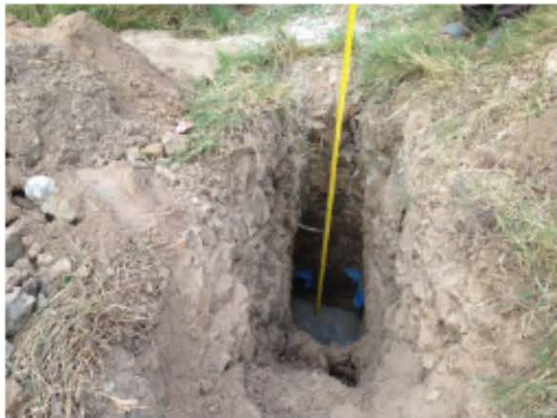
Test Pit No.12 (300 DIP Pipe found)
