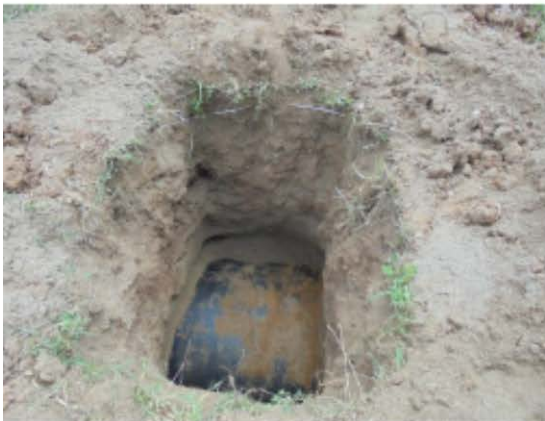
Test Pit No5 (1100DIP Pipe found)
