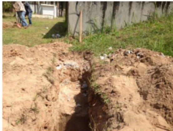
Test Pit No.6 (Existing Concrete found)
