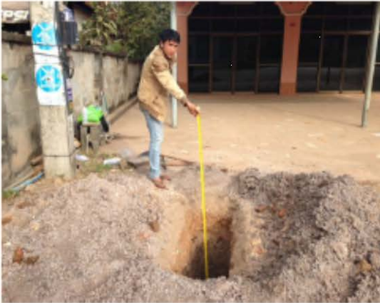
Test Pit No.13 (Pipe not Found, Over 2m-Dept found)
