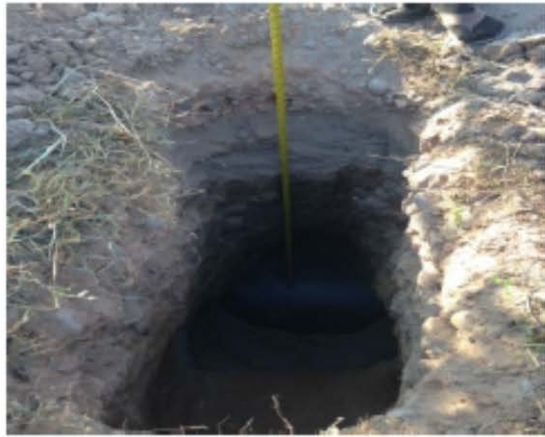
Test Pit No.20 (700 DIP Pipe Found)
