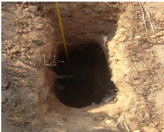
Test Pit No.19 (700 DIP Pipe Found) Found)
