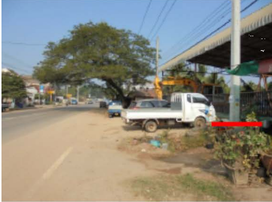
Test Pit No.11
