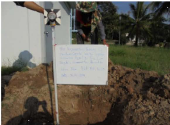
Test Pit No3(250DIP Pipe found) found)
