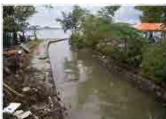
Untreated wastewater flow into the Bay (next to the night market at Than Nien Beach)
