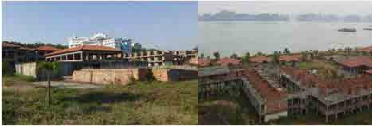
Unfinished accommodation (Tuan Chau Island)
