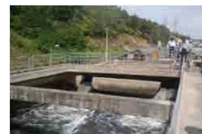
Bai Chay Wastewater Treatment facility
