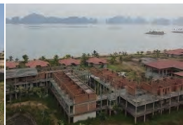
Unfinished accommodation (Tuan Chau Island)
