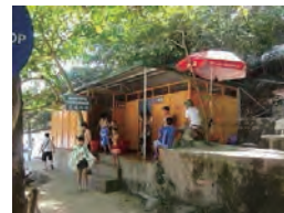
Poor condition of facility (Titop Island)
