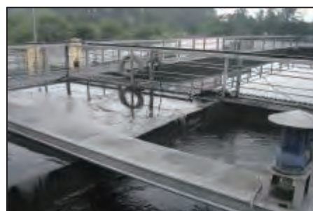
Photo 4 Coagulation Tank
