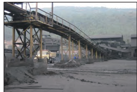
Photo 2 Coal Processing Yard
