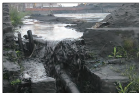
Photo 3 Wastewater Retention Pond
