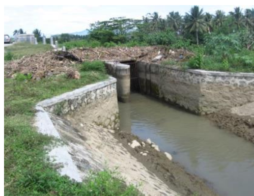
Note: Canal is clogged with mud and wood pieces from heavy rainfall. Photo taken in May 2014
