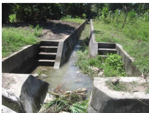
Note: Canal is clogged and water is not flowing. Photo taken in May 2014
