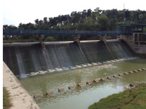
Photo 2: Weir constructed under the Project (Lanang)
