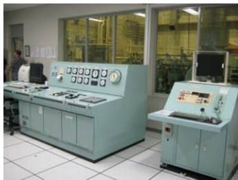
Diesel Engine Plant Simulator (BP3IP)
