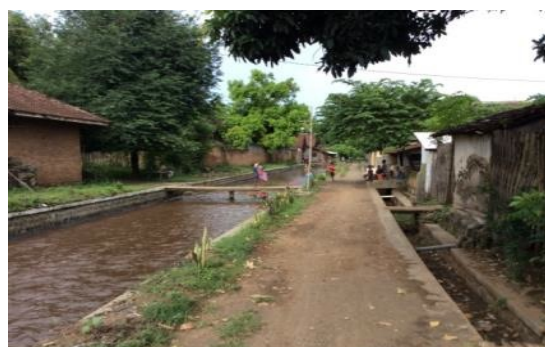
Photo 3: Road improved along the tertiary canal (Bajulmati)
