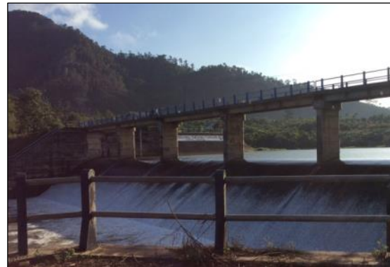
Dam Constructed under the Project (Batang Tongar)
