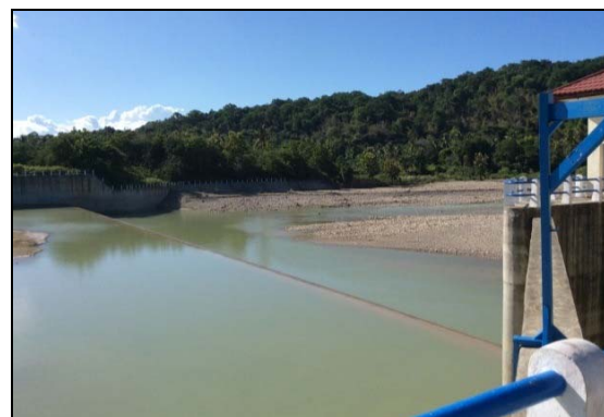
Constructed Weir of Malaka Weir Irrigation Project
