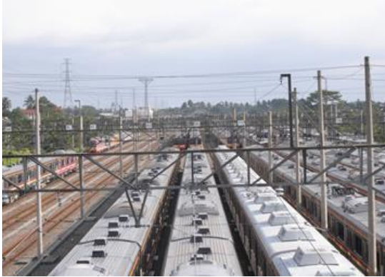
Photo 1. Commuter trains accommodated on the stabling tracks
