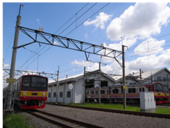
Depok depot (Inspection shed)
