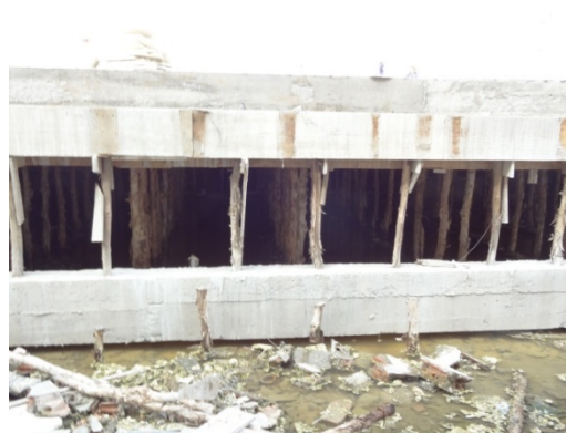
Photo 4: Melaleuca pole to sustain a concrete building
