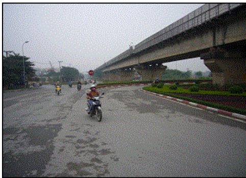
Thang Long Bridge South - Dike Road
