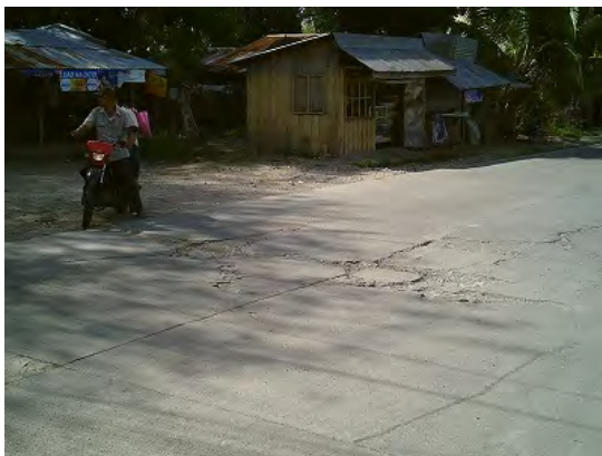
Damage on the Road Surface (Section 1)
