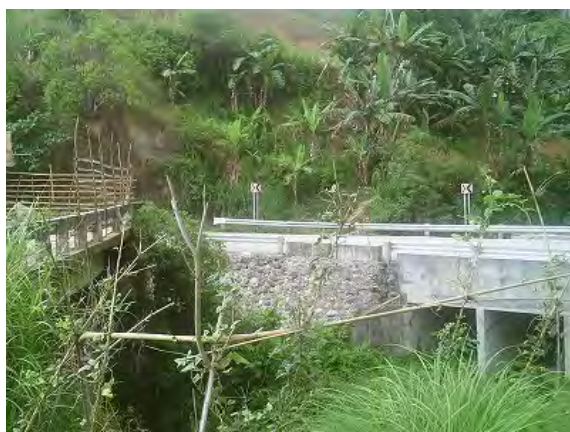
An old bridge on the left was abolished and the roads were rerouted with installment of a new box culvert (Section 2)
