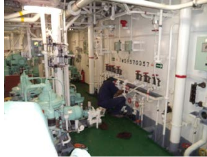
Photo 4: Inspection of the Engine Room
