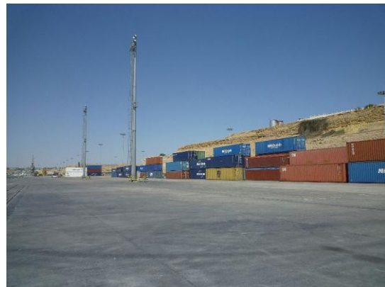
Photo 6 Yard of 3A Wharf
