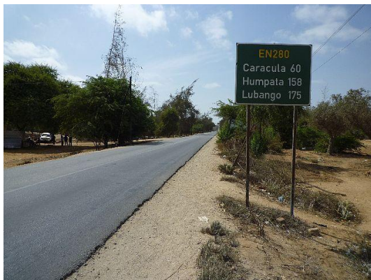
Photo 1 Highway to Inland in Namibe
