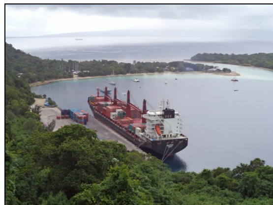
Main Wharf rehabilitated in this project and a cargo ship calling at the port
