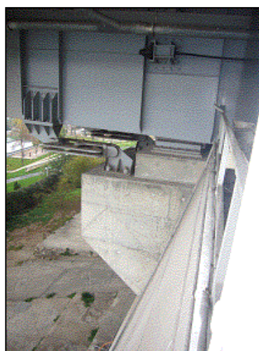
First Bosphorus Bridge Reinforcement of support at abutment
