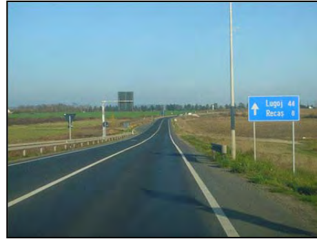
Timisoara - Lugoj Road (2-lane section)
