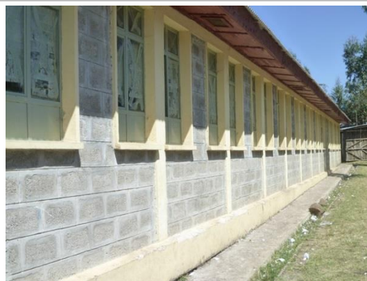
School buildings constructed in the Project
