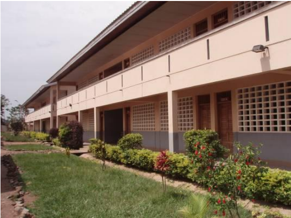
School Buildings Constructed in the Project
