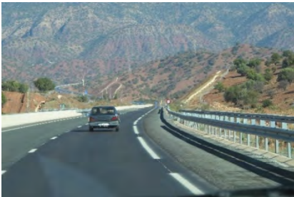
Motorway constructed under the project (the Argana to Ameskroud segment financed by the project)
