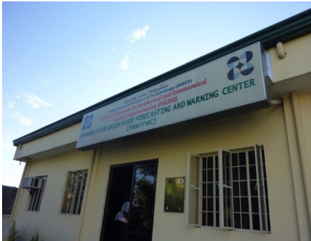
Photo 1: Constructed Pampanga Sub Center
