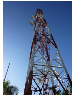
Photo 6: Constructed Telecommunication Steel Tower
