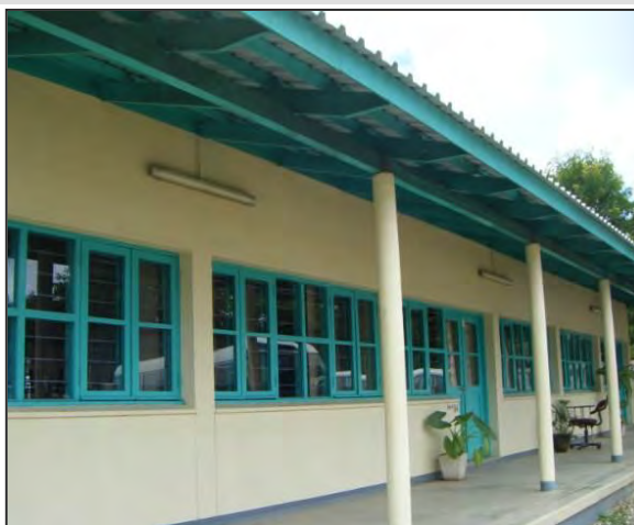
Constructed classroom (CFS Massinga)
