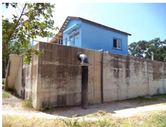
Welezo Reservoir developed in the project
