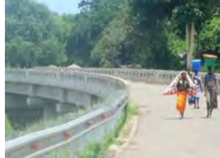
Constructed bridge (Chueza)
