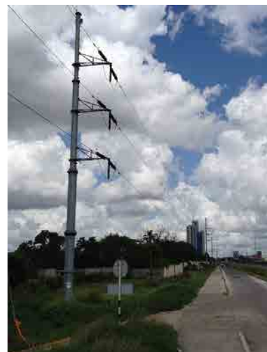
Photo 2: A transmission pole constructed in road reserves
