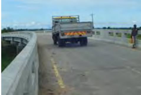
Replaced bridge (Cuacua I)
