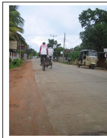
Road reconstructed by the Project
