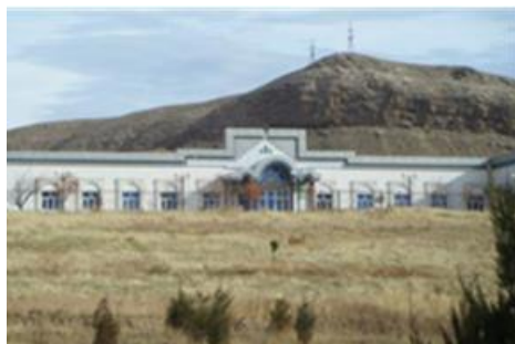
Constructed School near Darband Station
