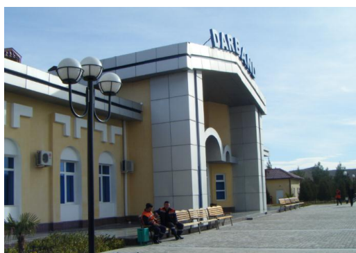
Newly constructed station (Darband Station)
