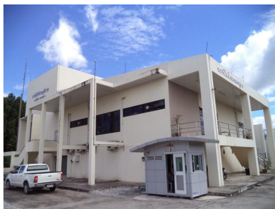
Sub-station constructed under this project (Nakhon Pathom Province)
