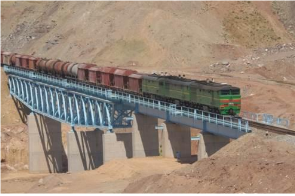
Constructed Bridge (Bridge No.5)
