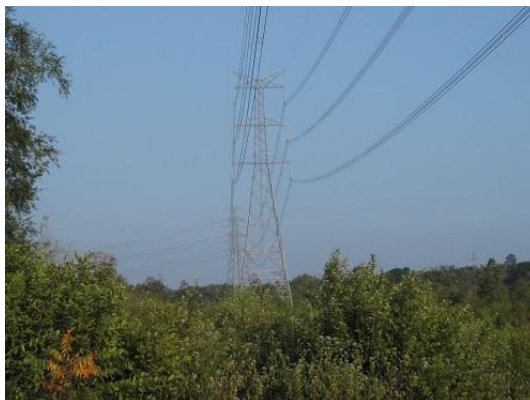
Transmission lines constructed under the project
