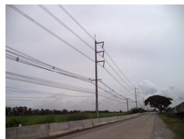
Transmission Line Constructed under This Project
