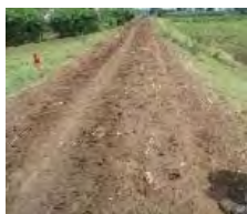
Dyke constructed during the Master Plan Study
