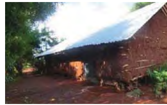
Heavy inundation of flood depth 1.2 M in Rekeke
