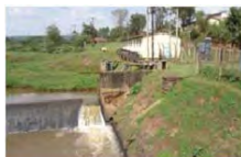
Water supply plant, binged on R. Gucha at Kegati
