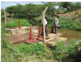
IWASCO water supply intake works
