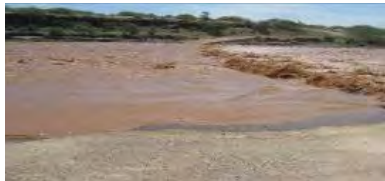
Submerged Gotu Bridge May 10, 2012
