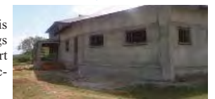
Disaster Centre under construction
