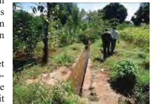
Channel for irrigation flow to reservoir
