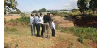
Survey on the eroded river bank at Eastern Maranja River
