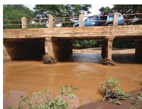
Bridge marking the boundary between lower and upper Lumi. The upstream side of the bridge is usually dry during the dry season. In wet season high flows from Mt. Kilimanjaro causes flash flooding
