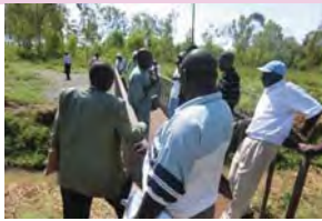
Observation of footbridge in Kamagaga village
