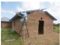
Reconstruction of houses
