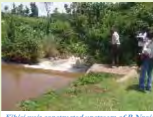
Kibisi weir constructed upstream of R Nzoia
