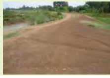
Dyke at Maumau in downstream of R Nzoia
