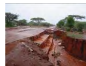
Gulleys as Factors in flooding
