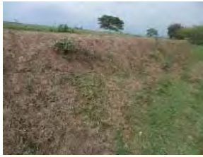
1.5 KM stretch dyke that has been constructed
