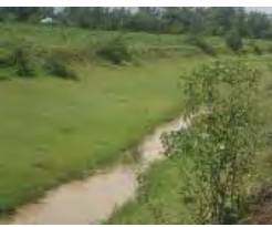
Spillway constructed adjacent to R. Nyando
