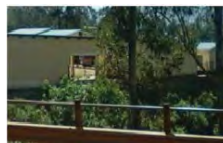
The condemned bus-park that was constructed next to R. Gucha
