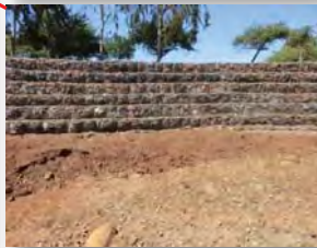
River Bank Protection using Gabion mattress
