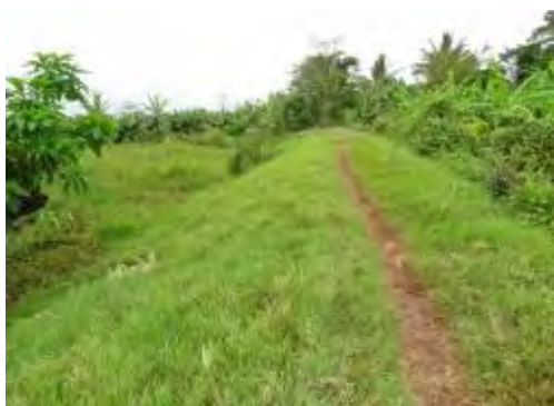
Photo 2.1.1 Embankment of the Canal-C
