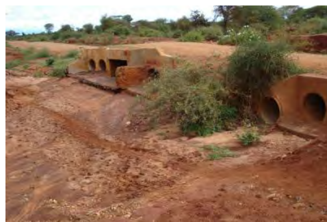
Bridge with pipe culvert installed at the dry up river crossing the road
