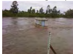
Automated River Gauging Station at Wath Onger
