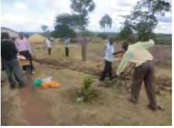
Installation process of rain gauge for CBFWS
