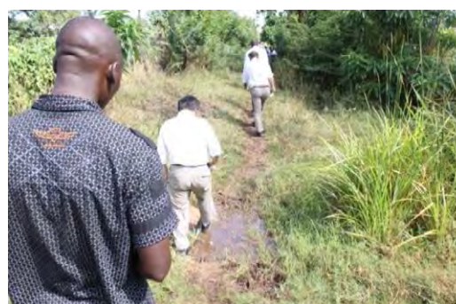
Photo 2.1.4 A Point of Artificially-destroyed Embankment (take agricultural water from Lumi R. of the left side on the photo and supply to the right side)
