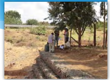
WRUA Monitoring and evaluation committee on site inspection during construction process
