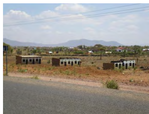
Houses were destroyed by flood
