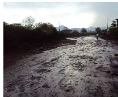
Road after flood Place: Isiolo Town
