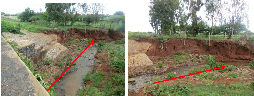
Photo 4.1.2 View of Downstream from the Crossing Point of Highway A2
