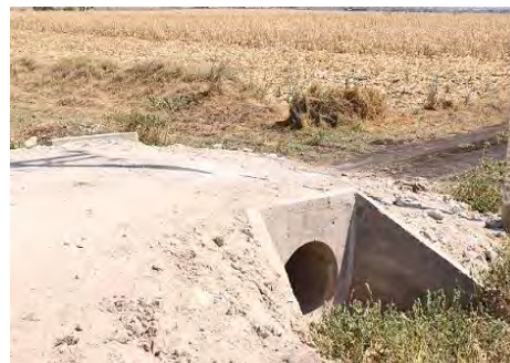
Culvert installed near the airport Place: Isiolo Town
