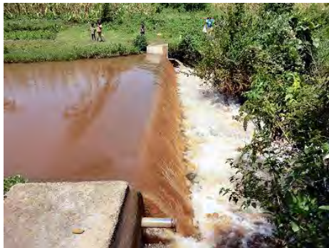
Check Dam (Example of Nzoia River)
