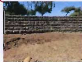
River Bank Protection using Gabion mattress
