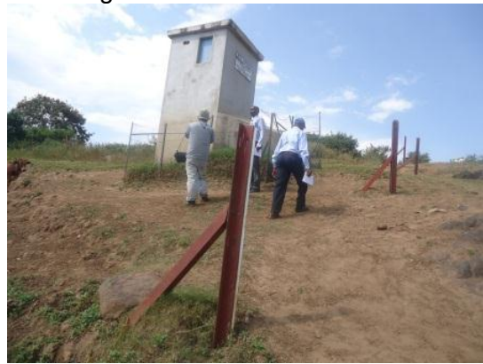
Water Level Gauging Station No.:1KB05 Observation River: Gucha Migori River Special Note: This is an automated gauge station that transmit data to WRMA Regional Office
