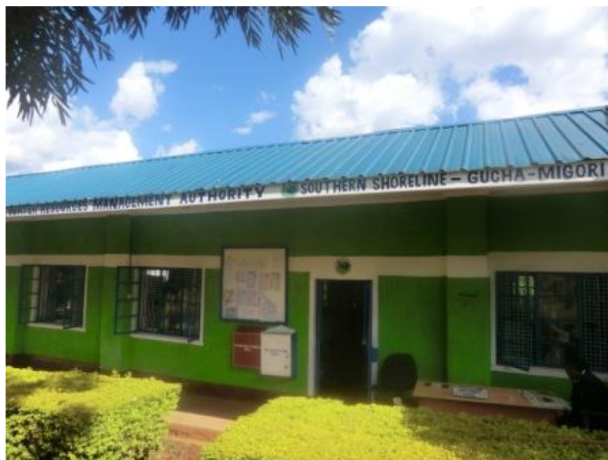
Figure 0.10 WRMA Southern Shoreline (Gucha Migori) Sub-Regional Office
