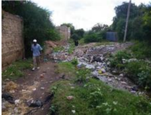
Many houses are built near the Merire River and the walls are encroaching river channel (upstream view)
