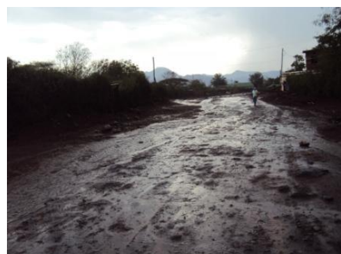
Road after flood (Place: Isiolo Town)
