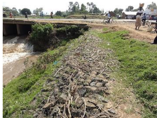
Example of river bank protection in Nzoia River
