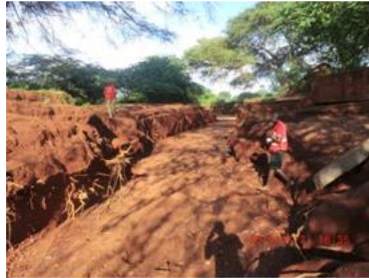
Wash out of land by bank erosion of seasonal river Place: Rekeke
