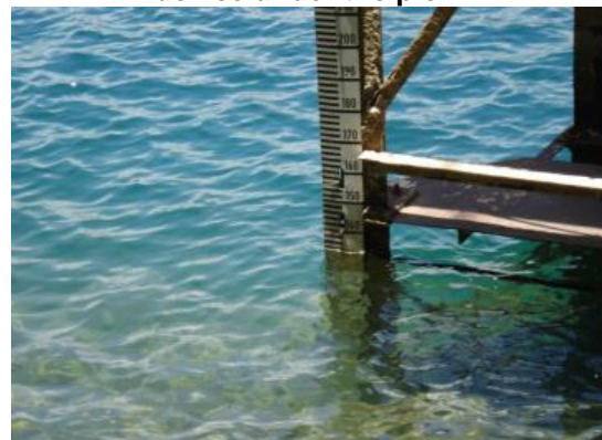
Water Level Gauging Station No.:3J12 Measure water level of Lake Challa.
