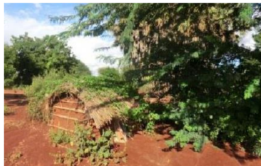
Toilet left as being buried by sedimentation by flood Place: Rekeke
