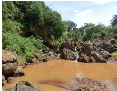
Status of water course after debris flow
