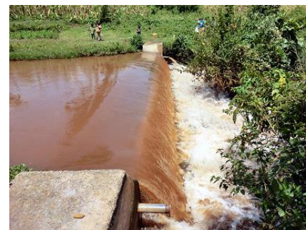
Check Dam (Example of Nzoia River)
