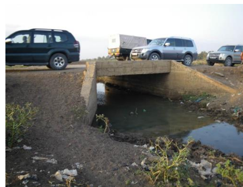
A box culvert bridge at the downstream end of the town of the Merire River (Downstream view)
