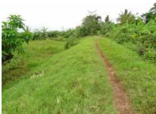
Photo 3.1.1 Embankment of the Canal-C
