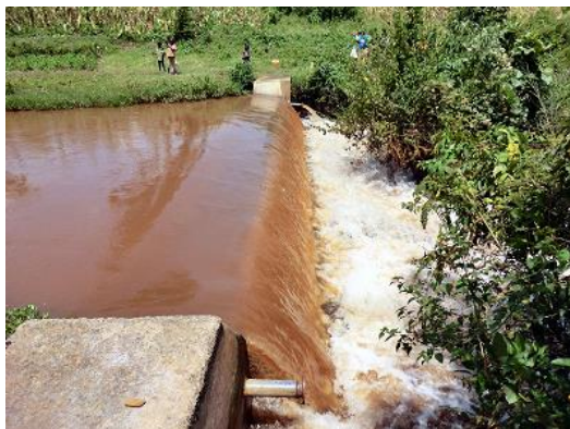
Example of check dam in Nzoia River
