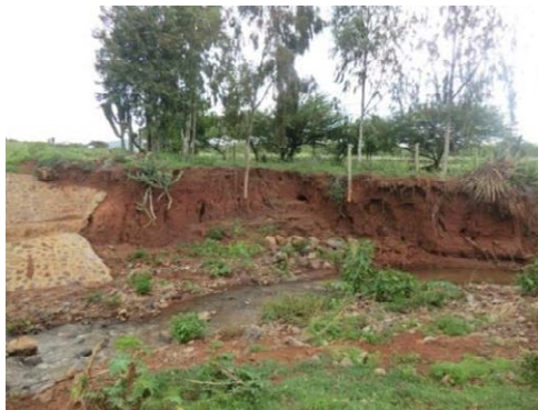
River bank erosion along Eastern Marania River (Place: Upstream of Isiolo River)
