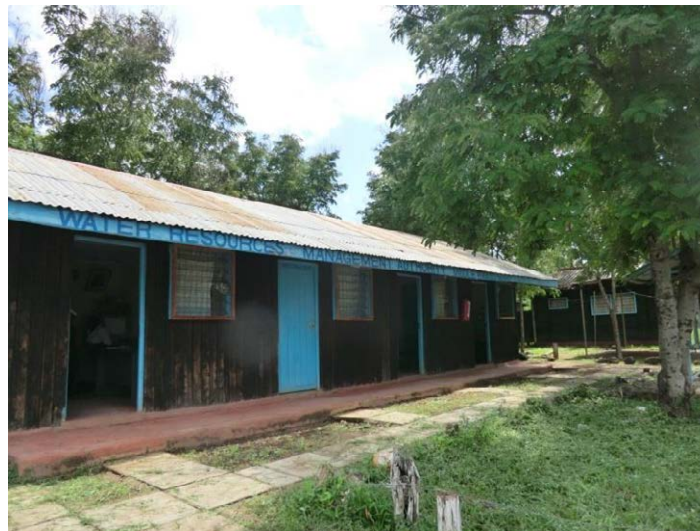
Photo 2.2.1 WRMA Middle Ewaso Ng'iro (Isiolo) Sub-Regional Office
