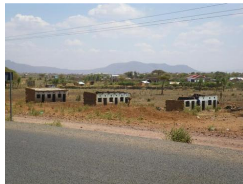
Houses were destroyed by flood
