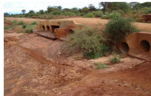
Bridge with pipe culvert installed at the dry up river crossing the road
