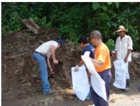
Figure-45 Putting Sand/Soil into Sandbags
