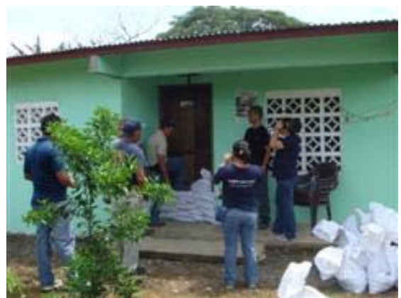
Figure-46 Setting Sandbags in front of Door
