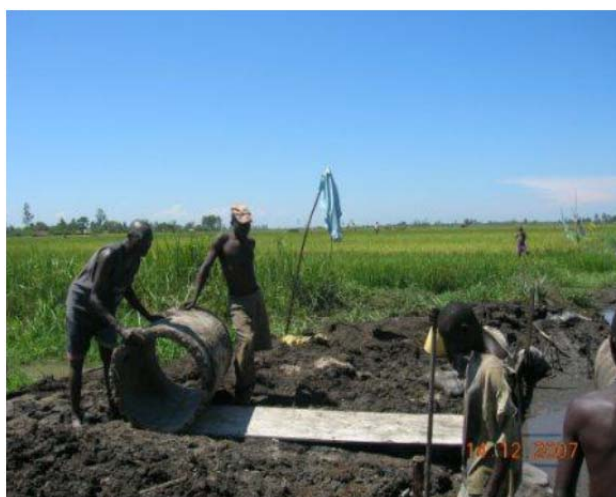
Figure-8 Community Repairing a Culvert to reduce Vulnerability
